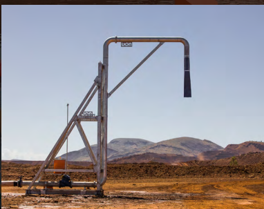
Standpipe Pump System
