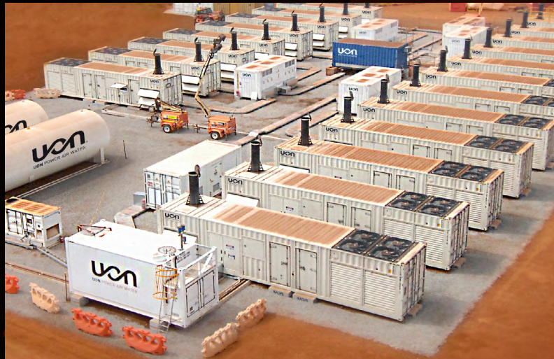
Rapid-Deployment 30MW Power Station
